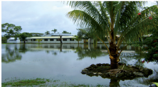
Flooding at Tupou high school, Vaololoa, 2013
