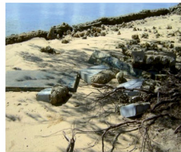
Coastal erosion, Lifuka Ha'apai, NEMO, MOW, 2009.
