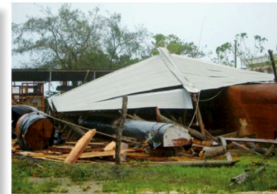
A house destroyed by Tropical Cyclone Rene, 2010, SNC Project Tonga, 2010
